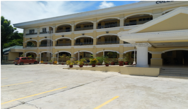
Figure 15. College of Law & Canteen Annex Site Photos
