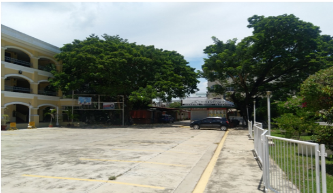
Figure 16. College of Law & Canteen Annex Site Photos
