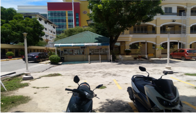
Figure 17. College of Law & Canteen Annex Site Photos
