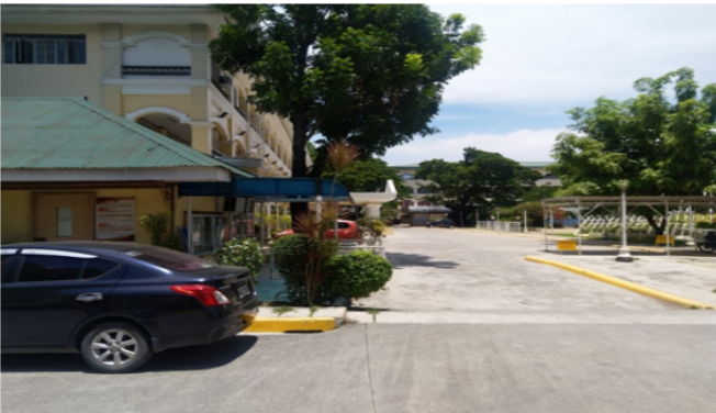
Figure 18. College of Law & Canteen Annex Site Photos
